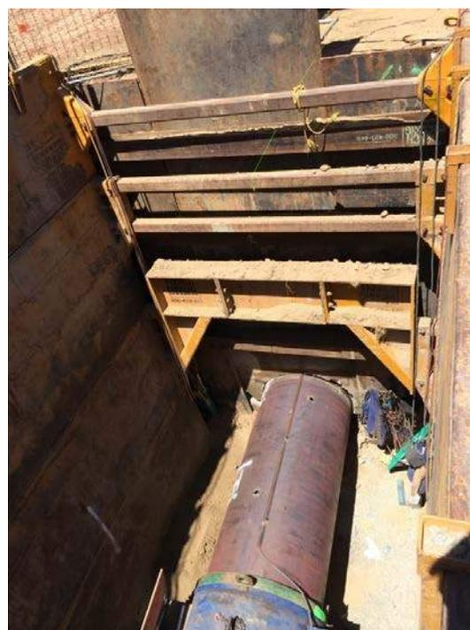
(b) Trench shields with auger boring
