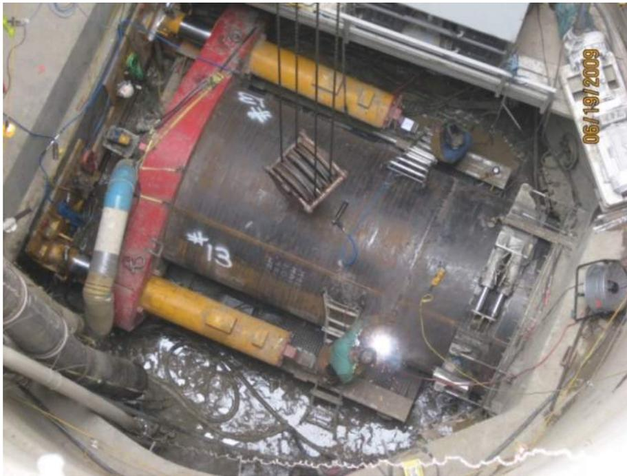
Figure A-8. Placing casing for jacking operation during microtunneling
