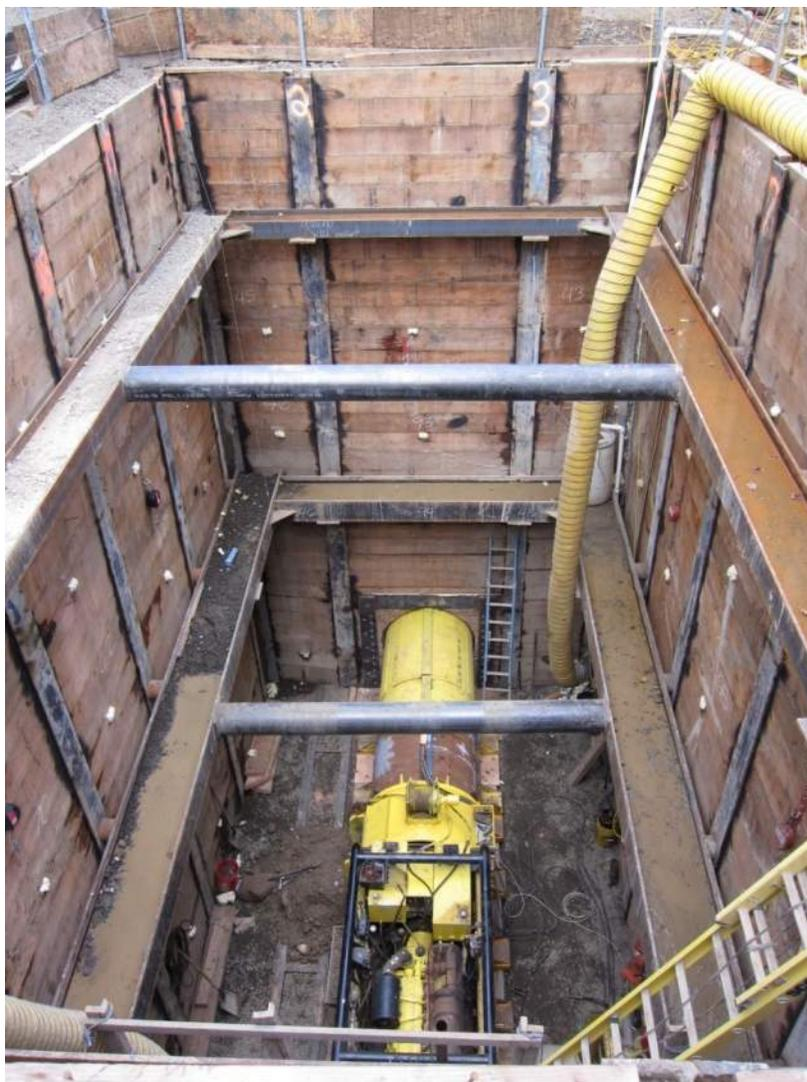
**Figure B-2. Trench shields supporting launch shaft excavation**
