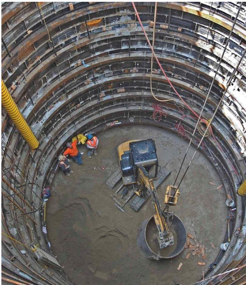
**Figure B-3. Typical liner plate shaft with ring beams and tie rods**
