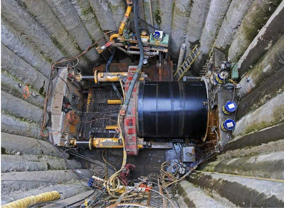
**Figure B-5. Typical secant pile shaft during the installation of a 108-inch ID casing)**
