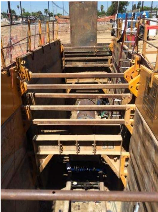
(a) Trench shields supporting shaft excavation
