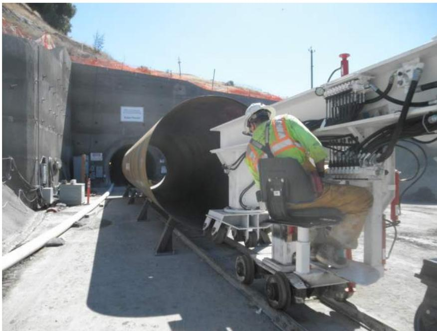
Figure A-11. Carrier pipe being transported into the tunnel
